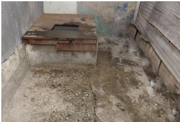
Image 5: Well elevated above ground level after the Project
